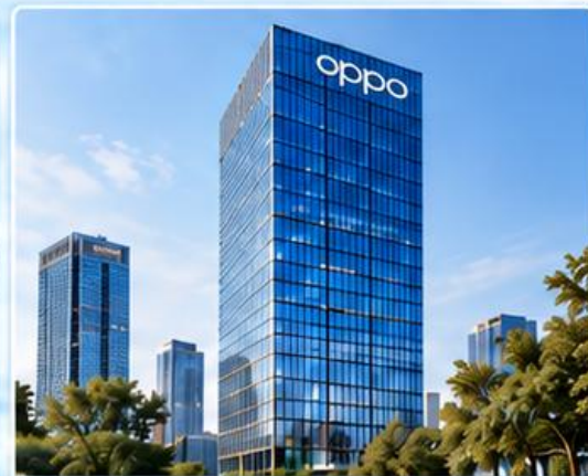
OPPO Tower China
